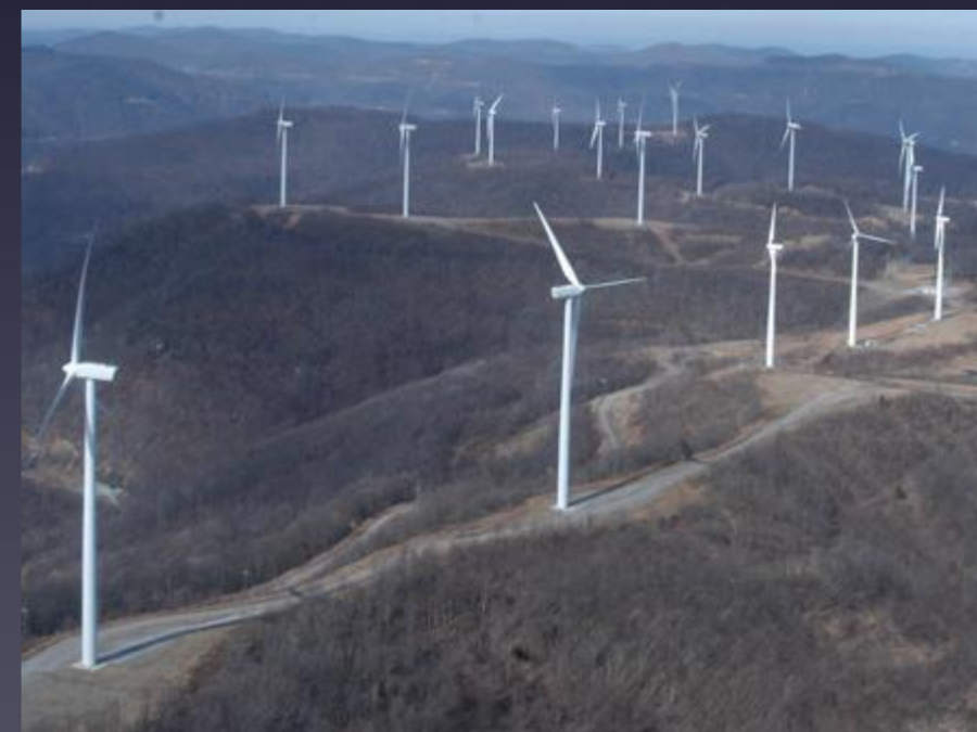
~18 wind turbines 3-4 MW each; 72 MW
