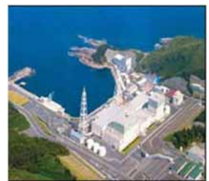
Shimane 3 Under Construction
