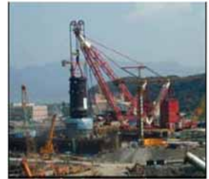
Lungmen 1 & 2 Under Construction
