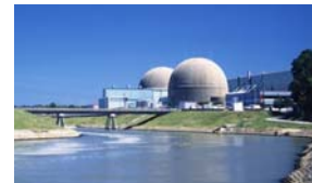
Surry Power Station
