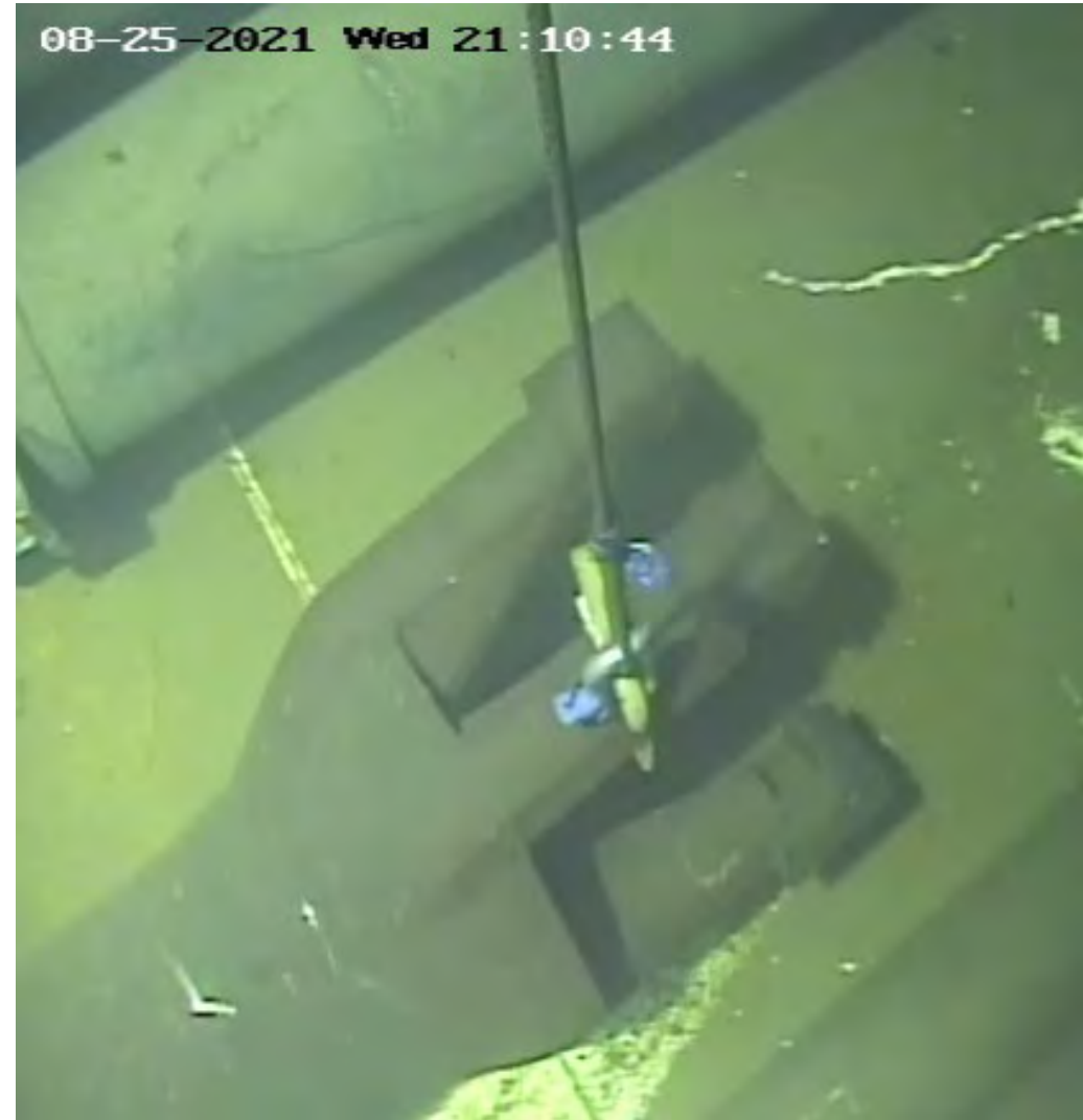
Jet Pump Inlet Riser Pipes are 13 feet long and segmented with specialty cutting tools
