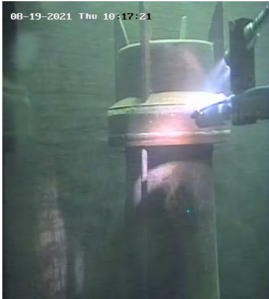
Jet Pump Diffuser removal
