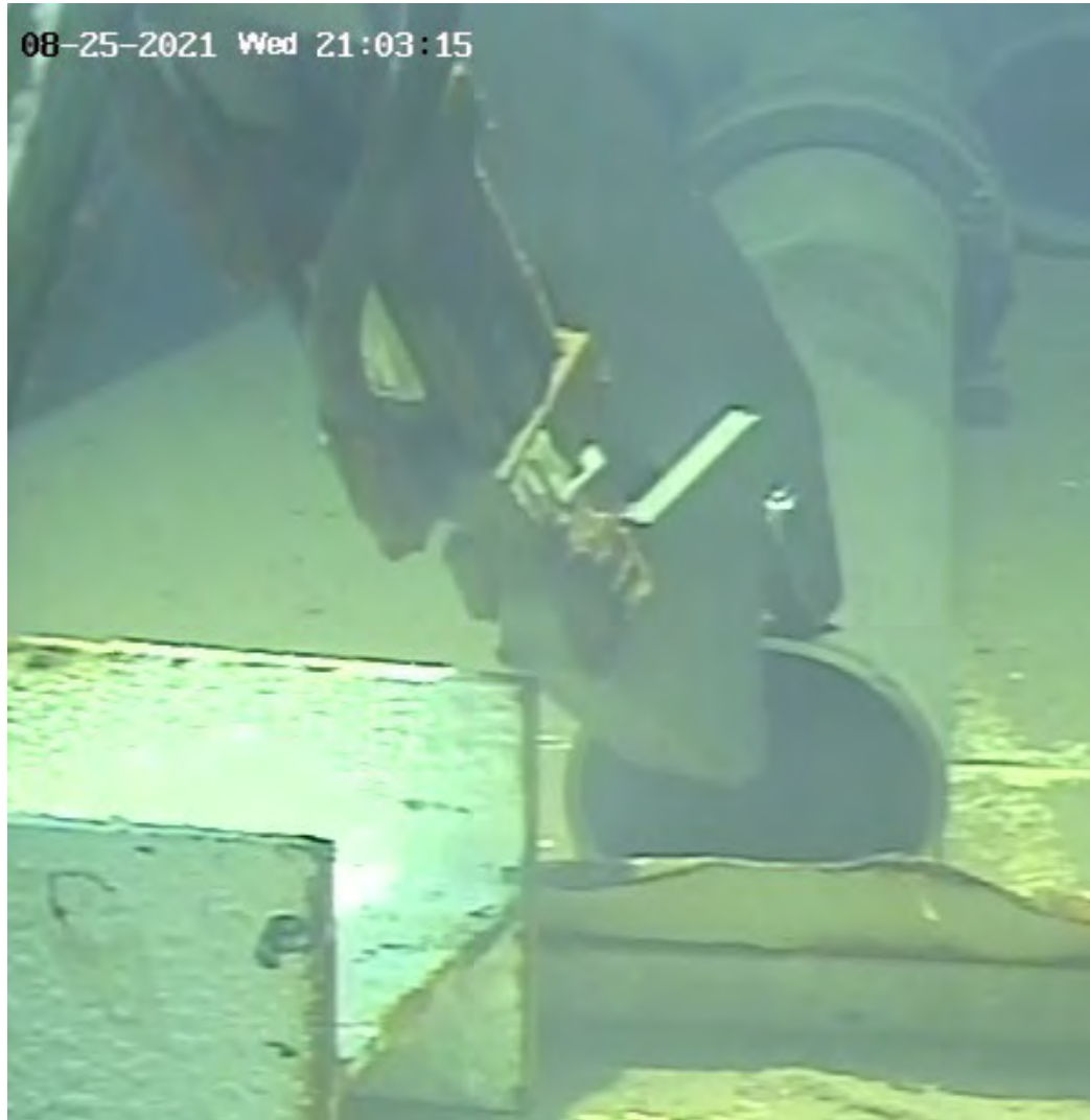
Jet Pump Inlet Riser Pipes are 13 feet long and segmented with specialty cutting tools
