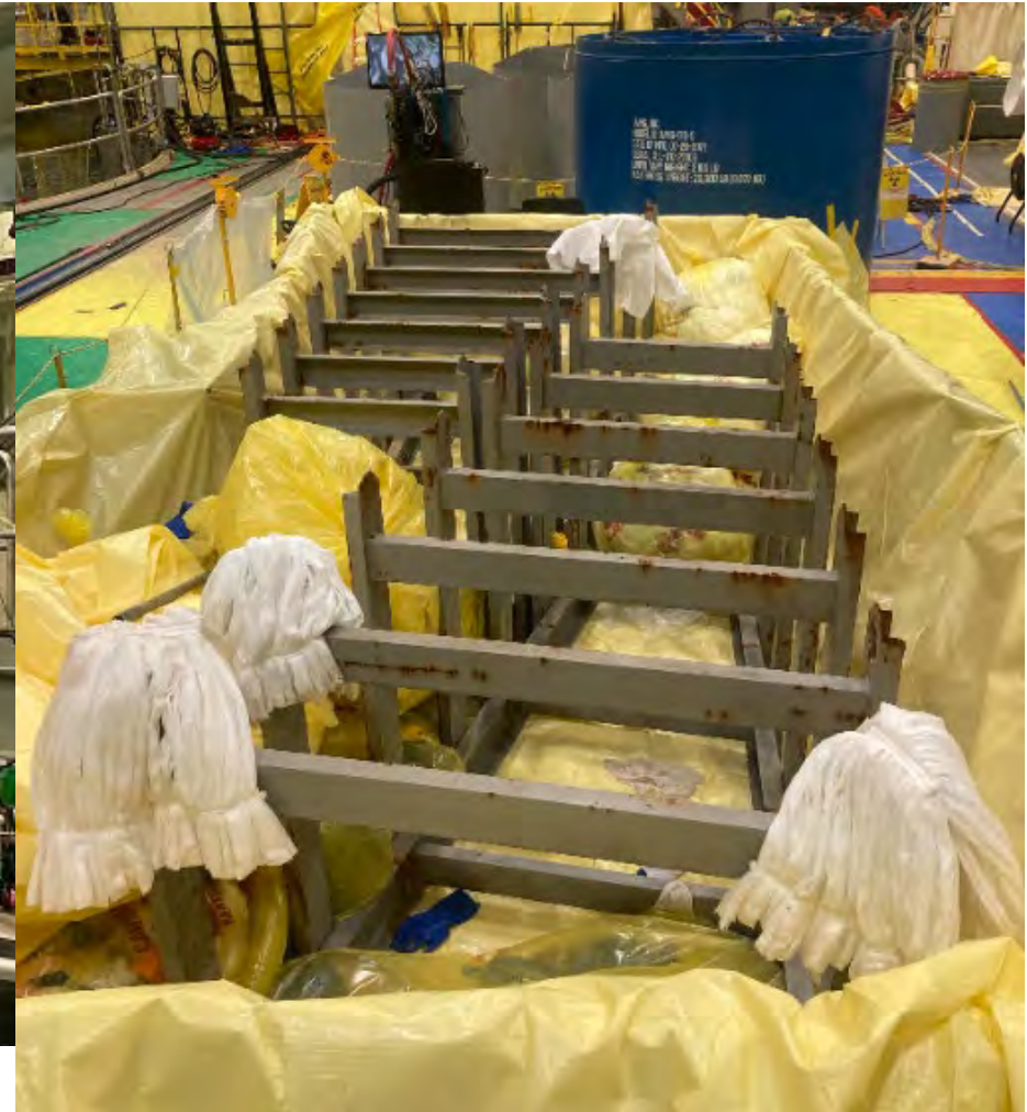
Racks decontaminated and packaged for shipment
