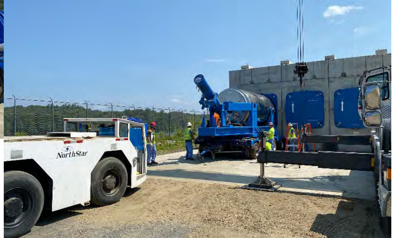
(5) Transfer into the HTS (Storage Vault)
