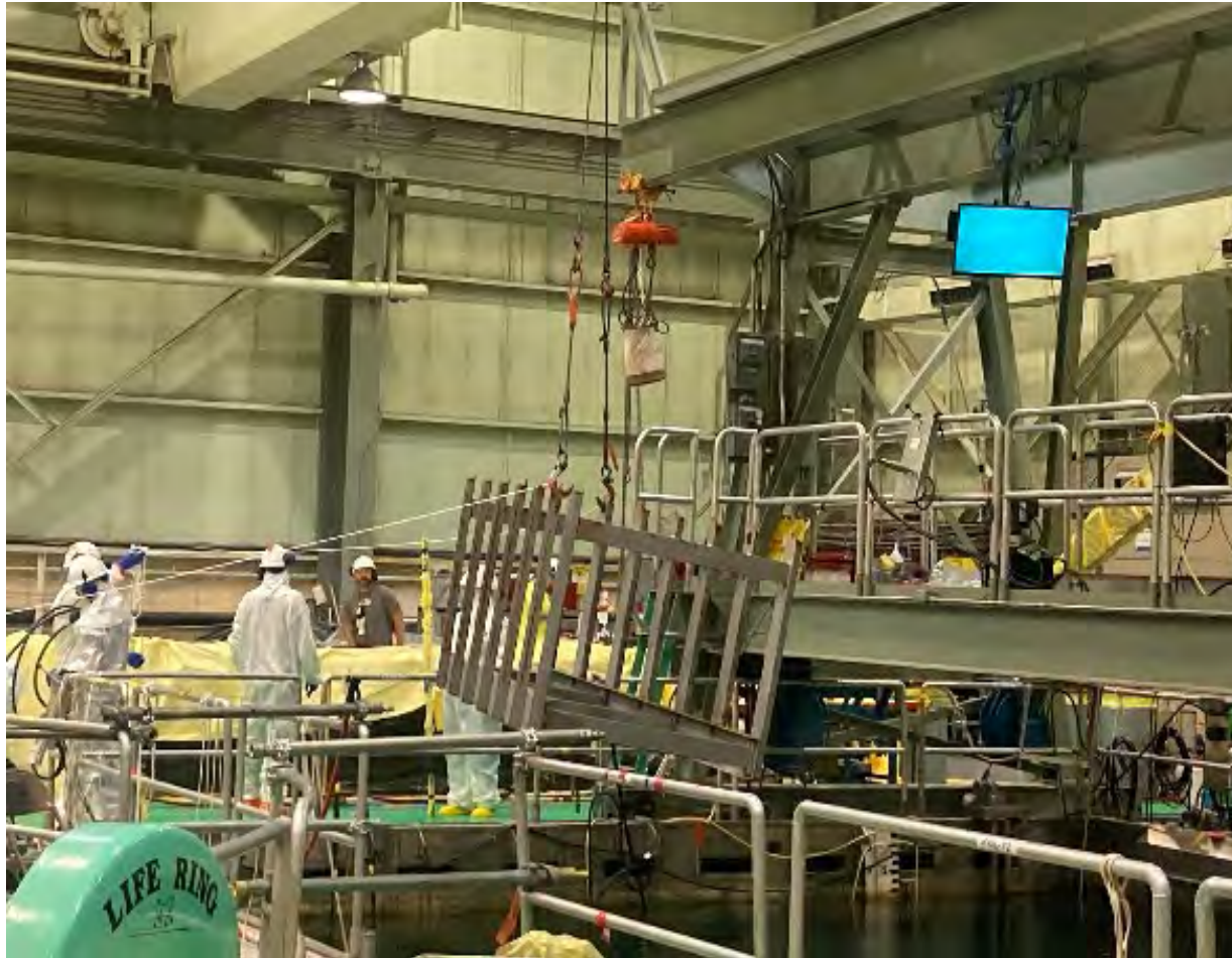
Removing the racks that once held Core Shroud segments in the Spent Fuel Pool, as they are no longer needed
