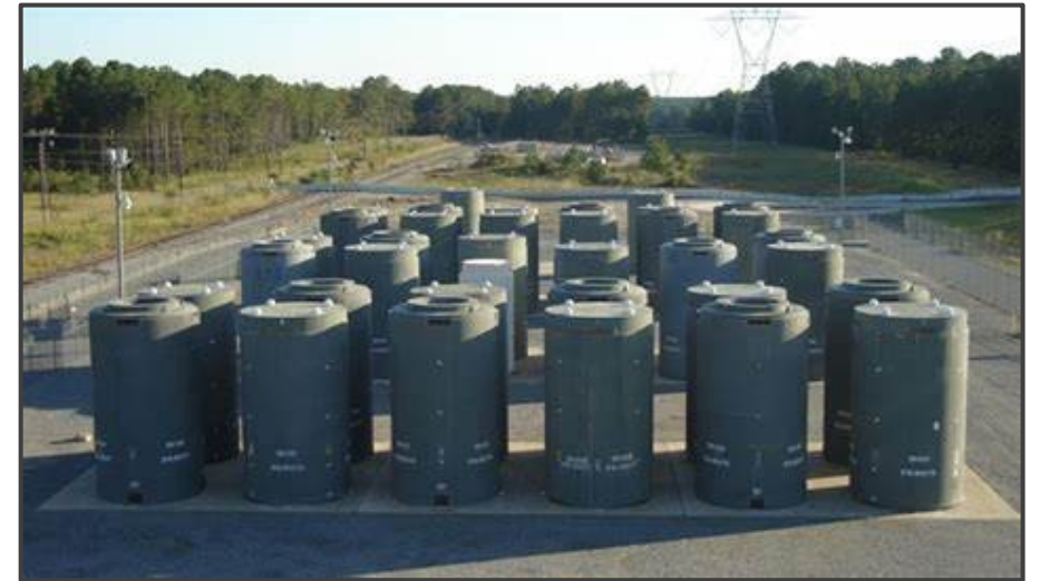
Holtec HI-STORM System (courtesy of Holtec International) ~ 4000 canisters being stored in U.S. at present
